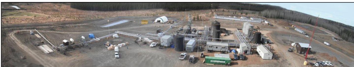
Aerial view of Blackrod SAGD Pilot Project during construction
